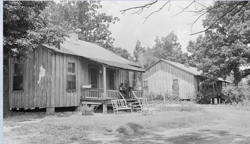
Workers sometimes lived in houses owned by the company.
