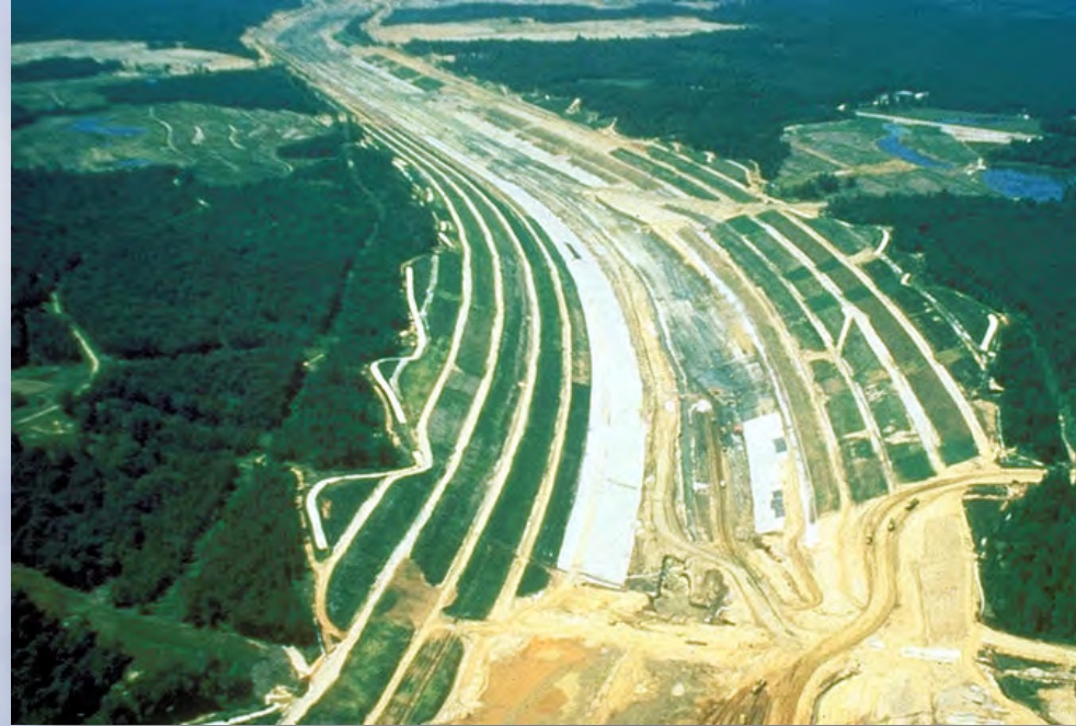
Construction of the Tenn-Tom Waterway in the 1980s.
