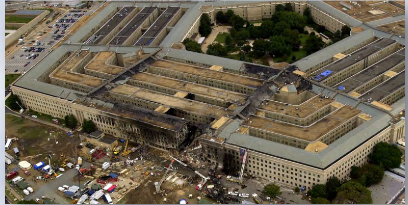
Pentagon damage on 9/11
