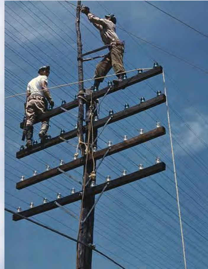
Workers install power lines for the TVA (1944).
