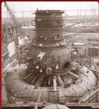
Above: Wheeler Dam, a TVA project on the Tennessee River, took three years to build. The dam was completed in 1936.
