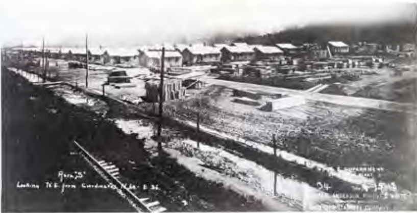
Erecting bungalows on 35th Street. In less than four months 1,724 houses were put up at an average rate of 18 per day
