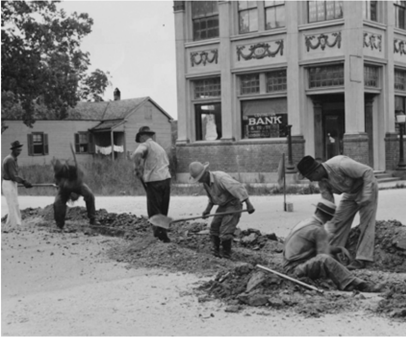
Left: WPA workers laying a water main in Madisonville in 1937. Bottom: Governor Earl Long.
