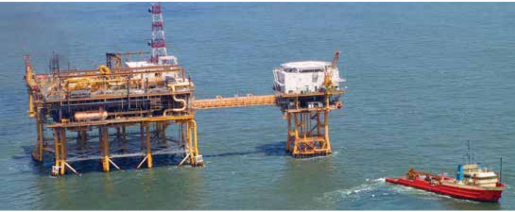
Left: This marine terminal is part of the Louisiana Offshore Oil Port (LOOP), which is the single-largest point of entry for crude oil coming into the United States by water. LOOP has offloaded over 11 billion barrels of foreign and domestic crude oil since it was built in the 1970s. Below: Canada, the United States, and Mexico are linked through the North American Free Trade Agreement (NAFTA).
