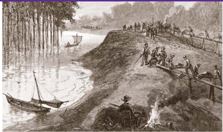
Above: Convicts working on the levee.
